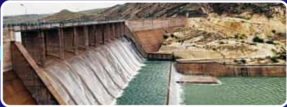
Darwat Gravity Dam-Sindh District Jamshoro.
