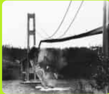
The collapsed, Tacoma Narrows Bridge.
