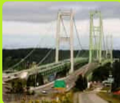
The newly built Tacoma Narrows bridges opened in 1950 (right) and 2007 (left). These bridges are built with much higher resonant frequencies.
