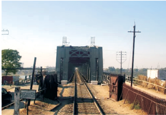
Kotri Railway Bridge
