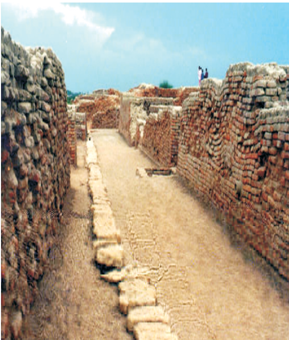
Fig 2.3 Houses built of baked bricks and the drainage system of Moen-jo-Daro
